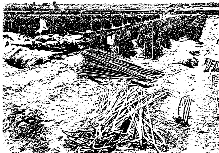
FIGURE 10.17. It is very important that frame parts and cages be arranged in an organized manner because several hundred cages will be erected during a one-week period.
